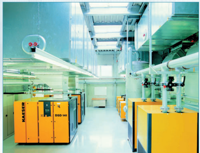
Figure 1. Compressed air system in a modern manufacturing plant. Comprehensive optimisation of the compressed air supply saves the company approximately € 70 000/yr in energy costs.
