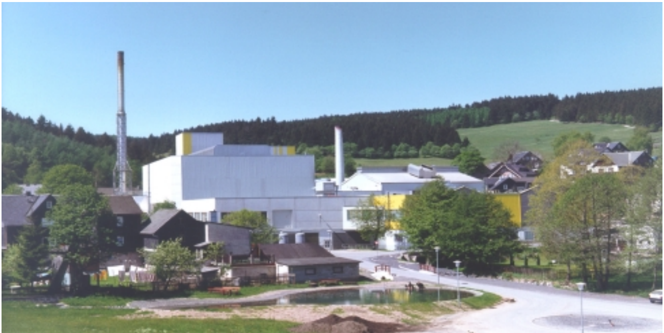
The Piesau glassworks, that has occupied this site since 1622, has now been modernized to the latest State-of-the-art. picture: Kaeser
